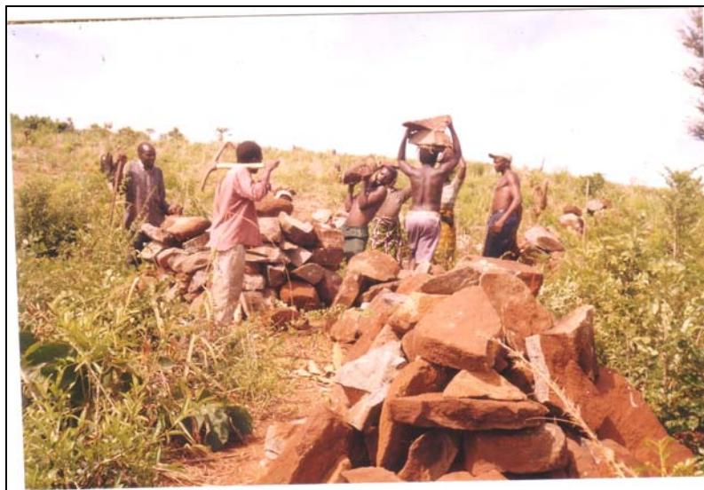
Photo 3: Kwafungo farmers busy collecting building material for constructing a classroom.
